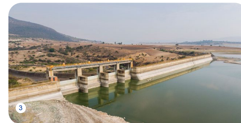
1 - CENTRAL NECAXA, FÉNIX - MEXICO 2 - CENTRAL LERMA, FÉNIX - MEXICO 3 - CENTRAL LERMA, FÉNIX - MEXICO
